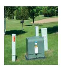
delay restoration work during an outage and create a serious safety hazard. We need at least 10 feet of clearance in front of the transformer (the side that is padlocked), as well as four feet of clearance on the other three sides.
